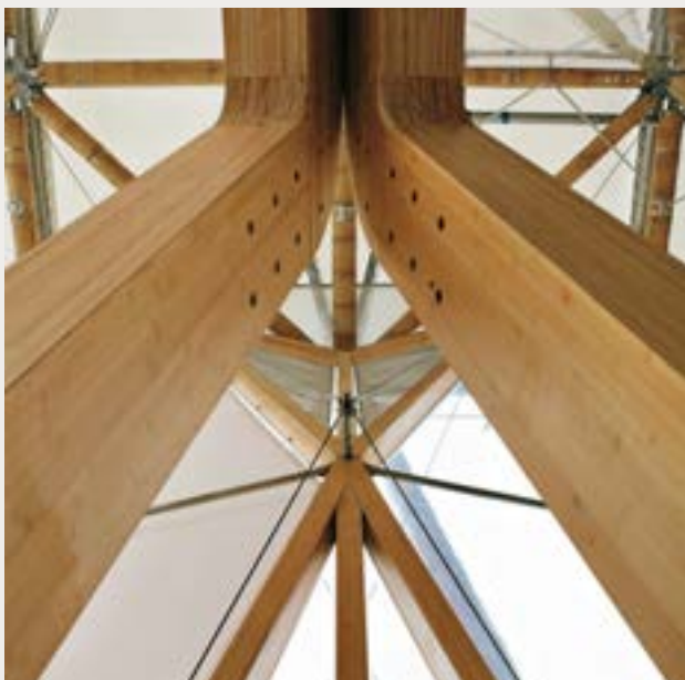
Custom structural bamboo beams
